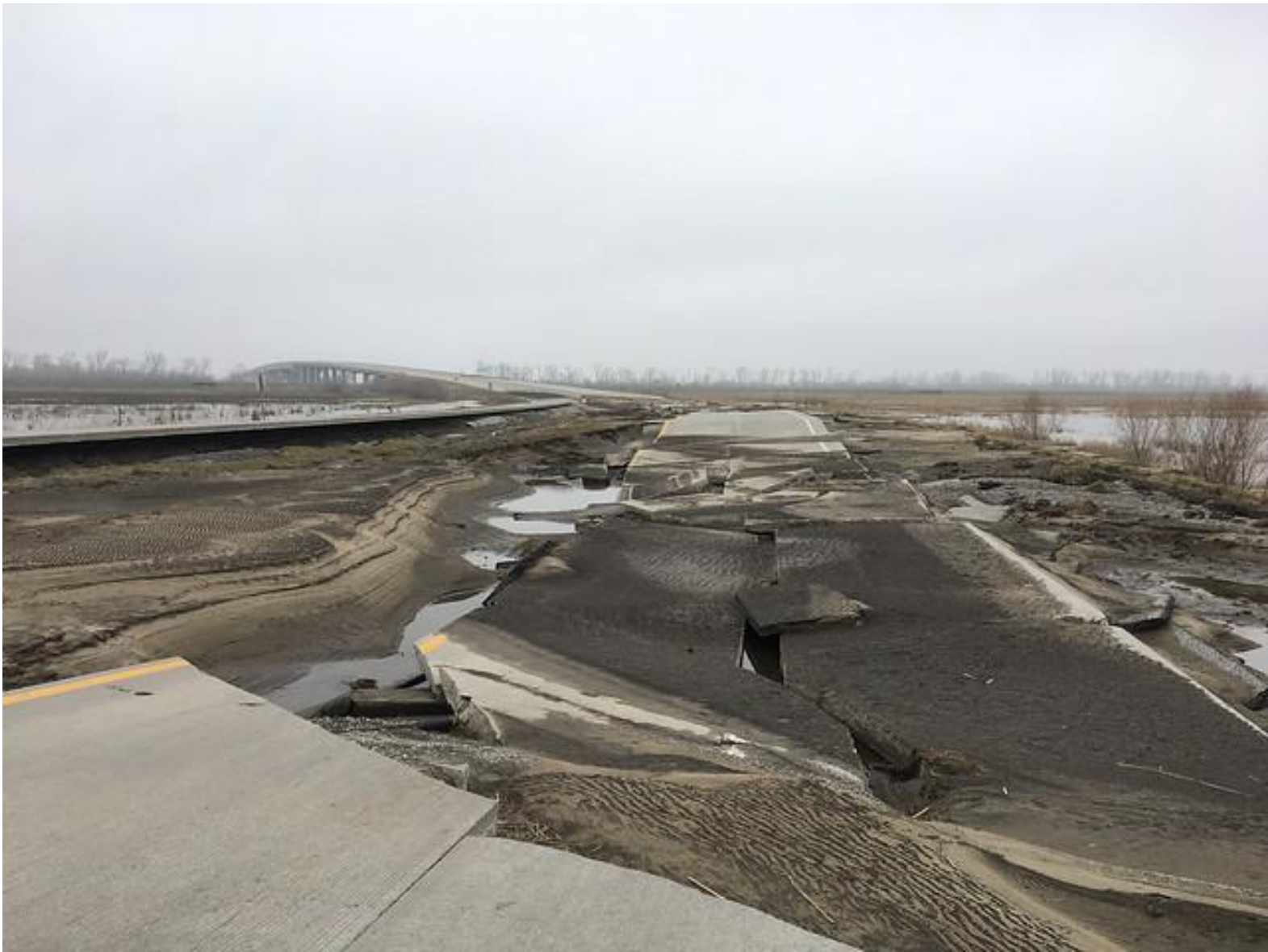
IDOT - 04/05/2019 - US 34 westbound looking west
