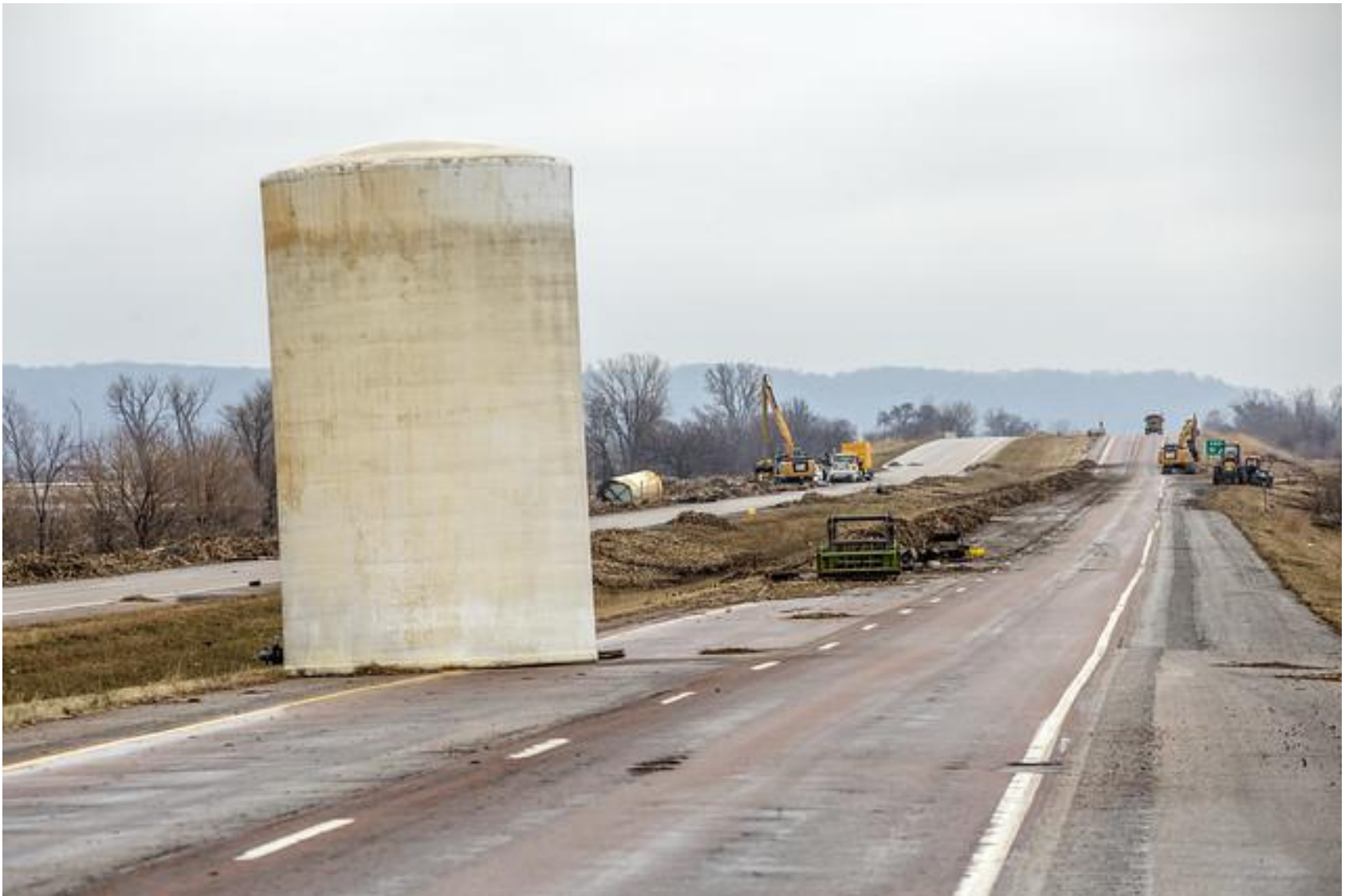
IDOT - 4/4/19 - I-29 between Hwy 34 and Hamburg
