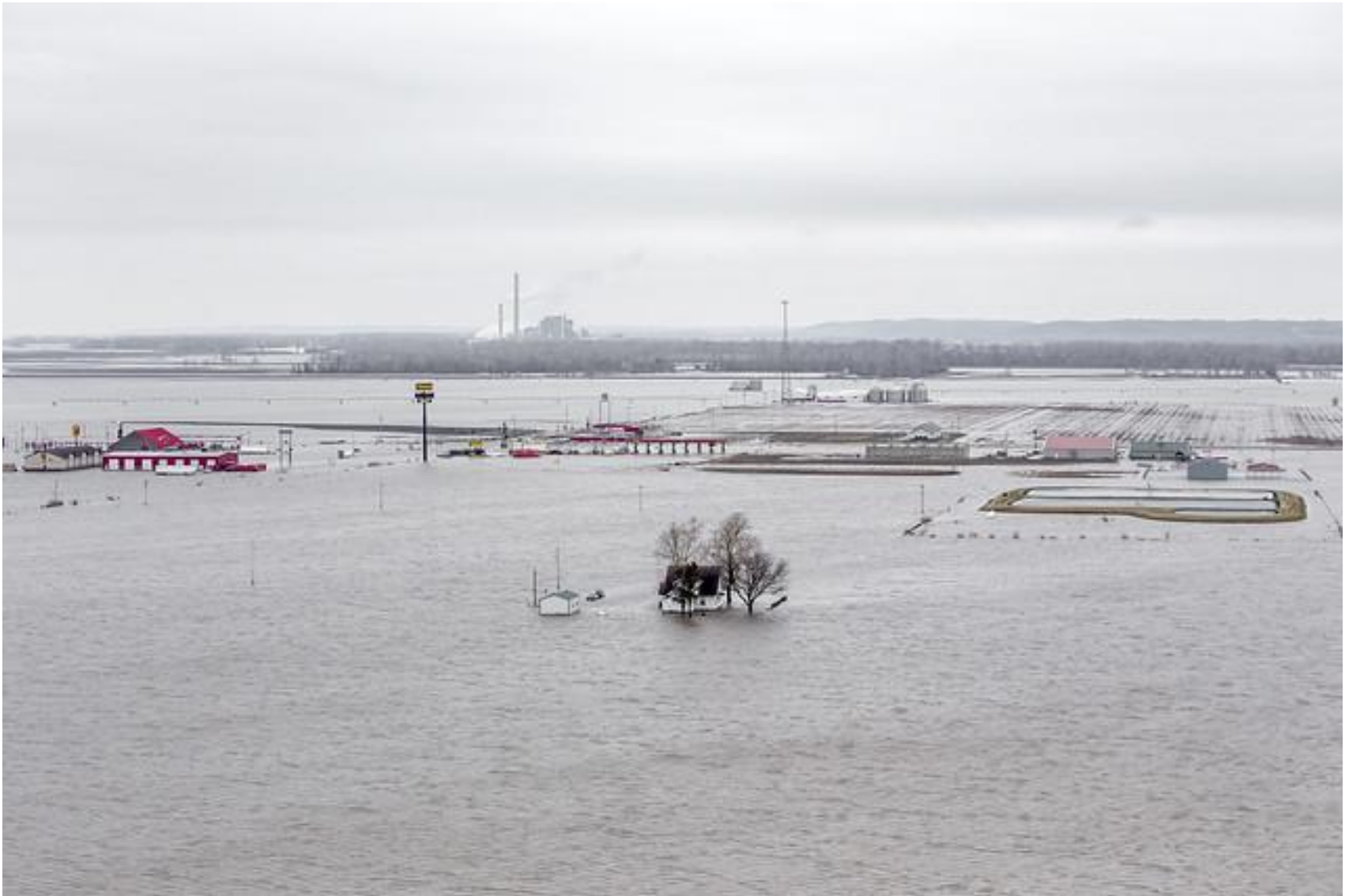
IDOT - 3/28/19 - I-29 at Iowa 2 interchange
